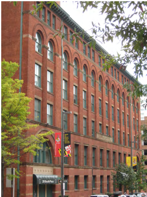
29 South Paca Street, the former Strouse & Brothers Building built in the late 1800s
