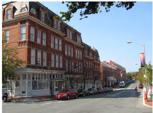
The Rieman Block (Lexington Street) is a historic collection of buildings listed on the National Register. Pascault Row can be seen in the background.
