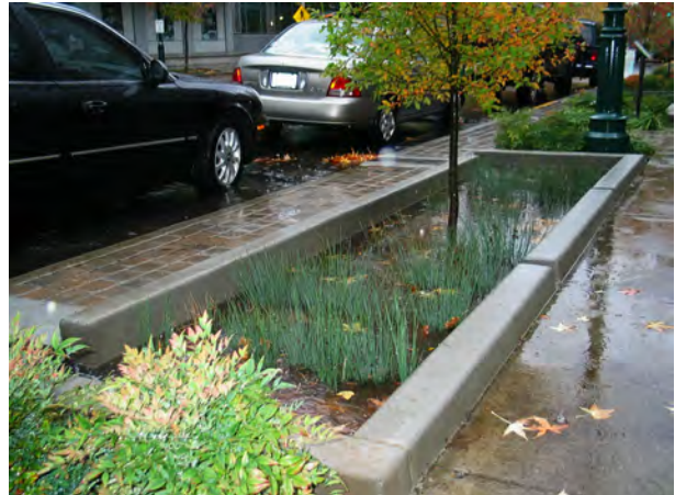
Stormwater inlet collects, filters, and detains run-off, Portland, OR
