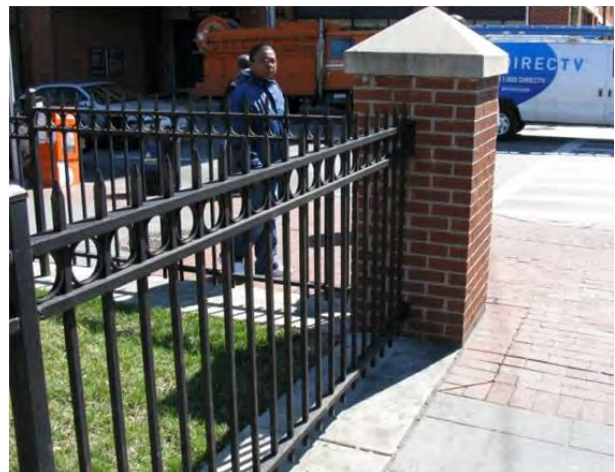
Example of existing secondary portal elements
