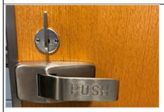
The is like a standard door lock and can be used by turning the thumb turn towards the door frame to lock the door (in this photo, the thumb turn would be turned to the left/counterclockwise.) The thumb turn can be turned away from the door frame to unlock the door (in this photo, the thumb turn would be turned to the right/clockwise.)
